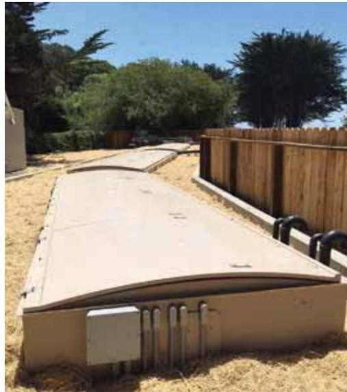
AX-Max<sup>™</sup> units, manufactured by Orenco Systems<sup>®</sup> of Oregon and obtained through PACE Supply of California. AdvanTex treatment systems use a fixed-film, attached-growth treatment process and are well suited to facilities receiving seasonal flows – such as parks, rest areas, and campgrounds.
