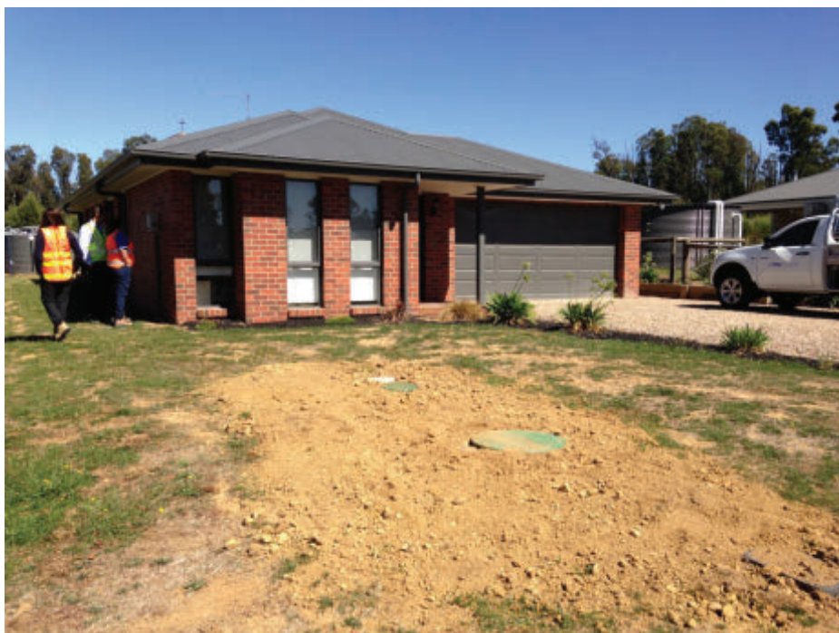
The Orenco STEP package includes a buried, watertight tank.
