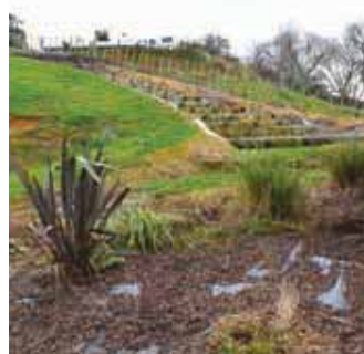
Above: A rock outfall provides final aeration of effluent in Piopio. Photo by InnoFlow Technologies
