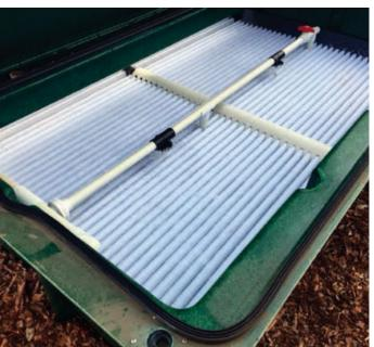
Treatment media in the AdvanTex AX100 is a uniform, engineered textile, which is readily serviceable and allows significantly higher loading rates than traditional recirculating gravel or sand filters. Photo by ENVIRA Holdings
