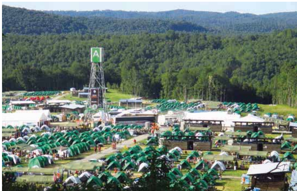
The AdvanTex Graywater Treatment Systems in place at the Summit Bechtel Reserve are an important part of the facility's overall sustainability. AdvanTex technology is known for its low energy use and for effective treatment, even with the highly variable flows common to camping areas. Photo by Biohabitats, Inc.
