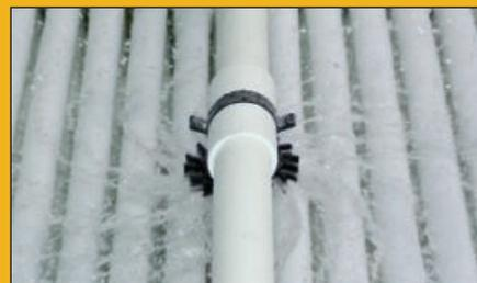
High-quality, low-horsepower pumps micro-dose the treatment media at regular intervals, and proprietary spin nozzles efficiently distribute the effluent, optimizing treatment.
