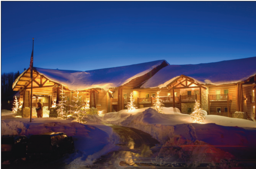
Daniels Summit Lodge in Utah, attracts outdoor enthusiasts year-round. This beautiful mountain location installed an AdvanTex ® wastewater treatment system to accommodate a restaurant expansion. Photo courtesy of Daniels Summit Lodge.
