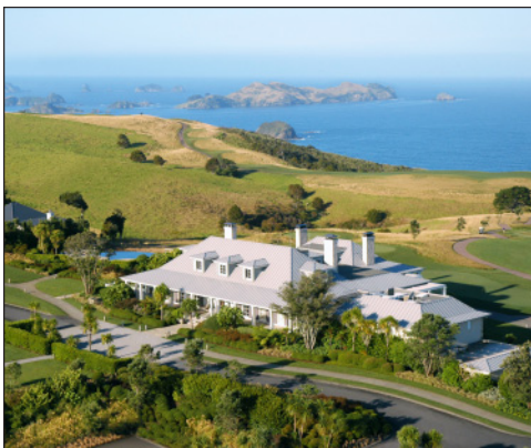
Kauri Cliffs, an award-winning Relais & Chateaux golf resort in New Zealand, replaced its failing activated sludge plant with an AdvanTex system, minimizing unpleasant odors in the process. Photo courtesy of Kauri Cliffs.
