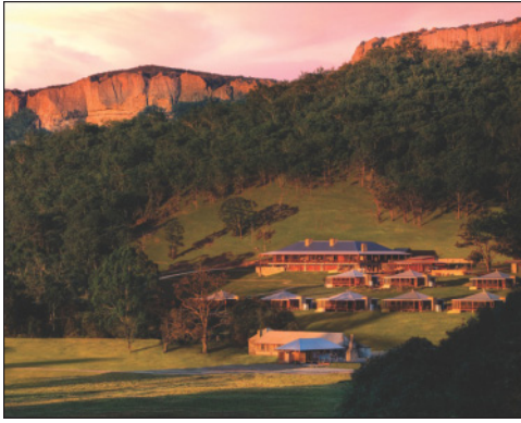
Emirates Wolgan Valley Resort and Spa, an eco-resort in Australia, chose a low-impact AdvanTex system to meet the needs of its environmentally sensitive site. Effluent is disinfected and used for irrigation. Photo courtesy of Emirates Wolgan Valley Resort and Spa.
