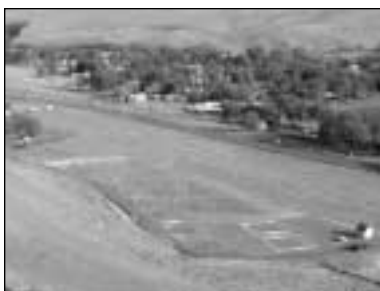
Aerial view of Starbuck, Washington and its AdvanTex® Treatment System.
